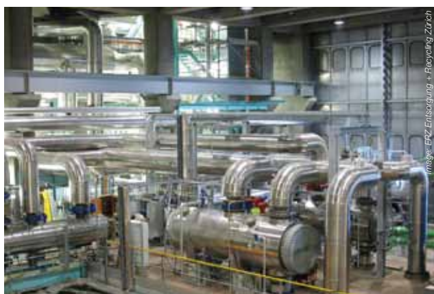
Feeding hot water into the district heating networks: heat condensers in the new Aubrugg wood-fired cogeneration plant.
