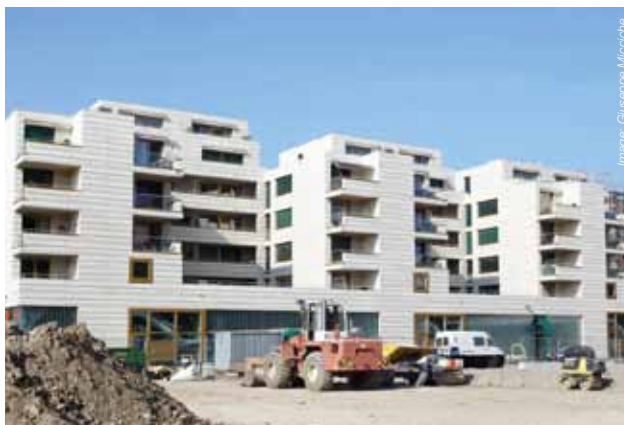
Living in compliance with the guidelines of the 2000-watt society: the Zurlinden society's residential complex on Badenerstrasse.
